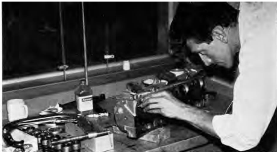
ABOVE —Milt Schornack, Royal's top drag racing expert, gives particular attention to the valve job during the Bobcat installation, saving time on the subsequent blue-printing operation phase of the program.
